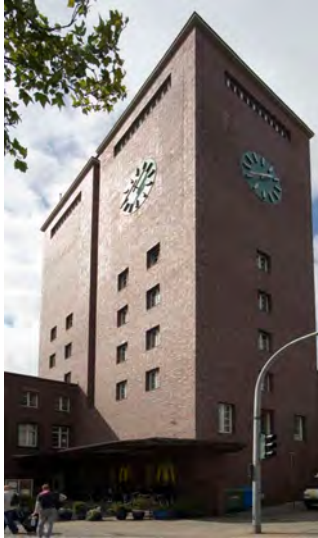
The station in Oberhausen
